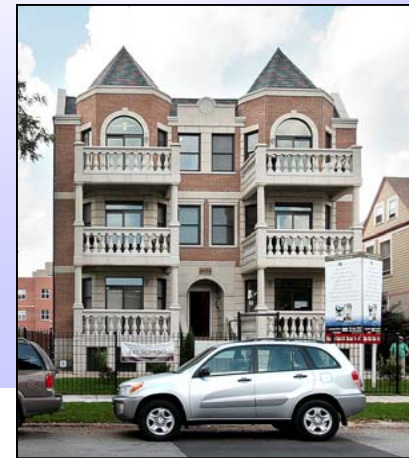
New Construction 4624 S. Greenwood
