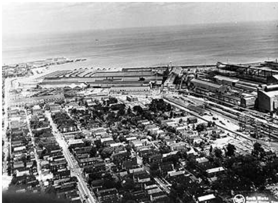
Arial View of US Steel Site
